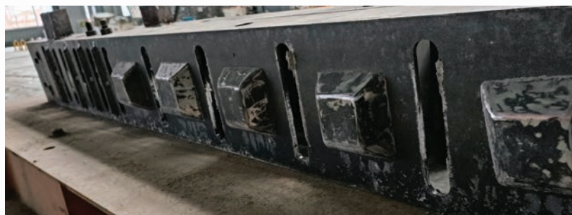
Picture 2: Shear key replacement for rough surface process
