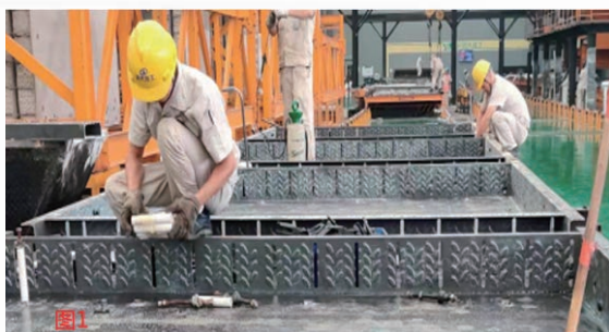
Picture 1: one-off moulding of rough surface
